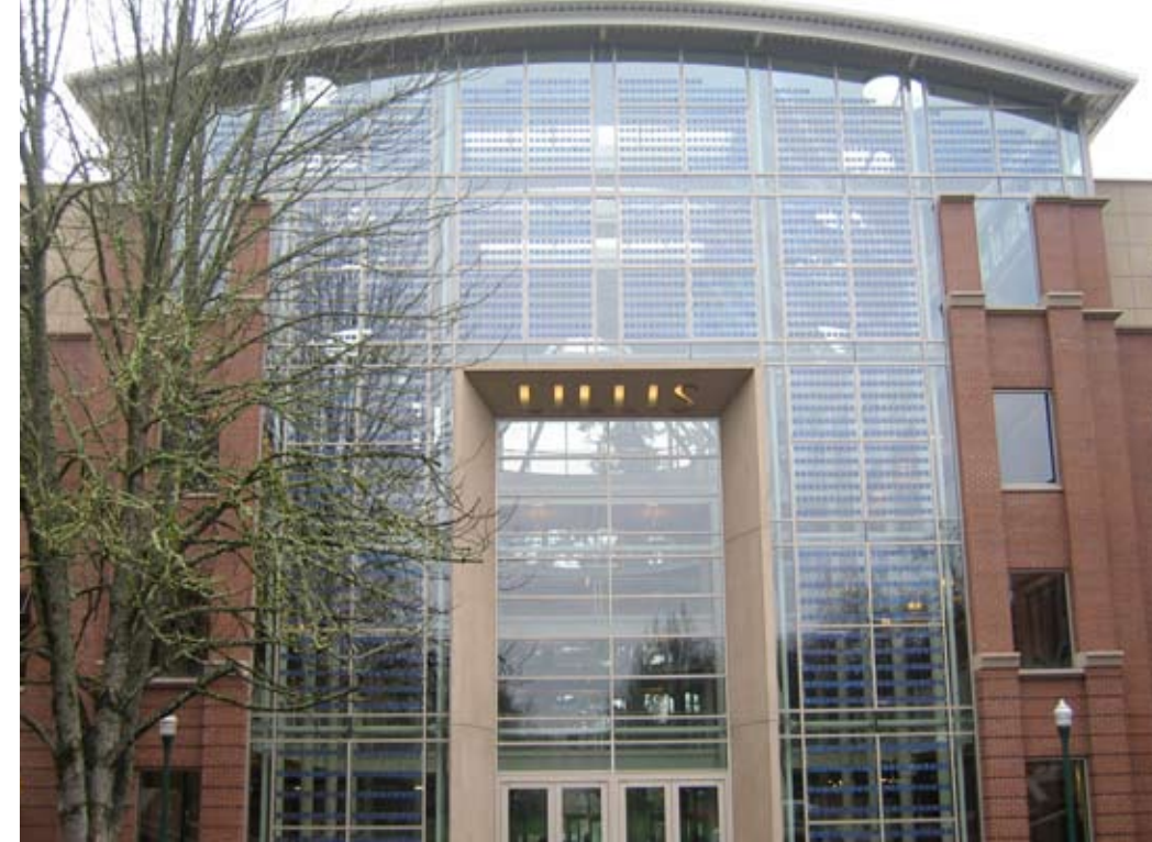
The University of Oregon's Lillis Business Complex is a LEED-certified building.
