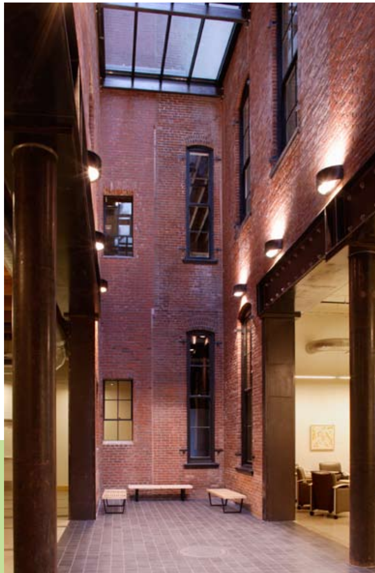
The University of Oregon's White Stag Block is up for LEED Gold certification. The facility harvests storm water from the building, treats it on site, uses greywater in its , and features low-flow fixtures; the entire system reduces city-supplied-water use in the building by 86%.
