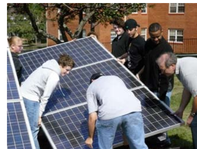
Students at Mercyhurst College help install solar panels on the campus.
