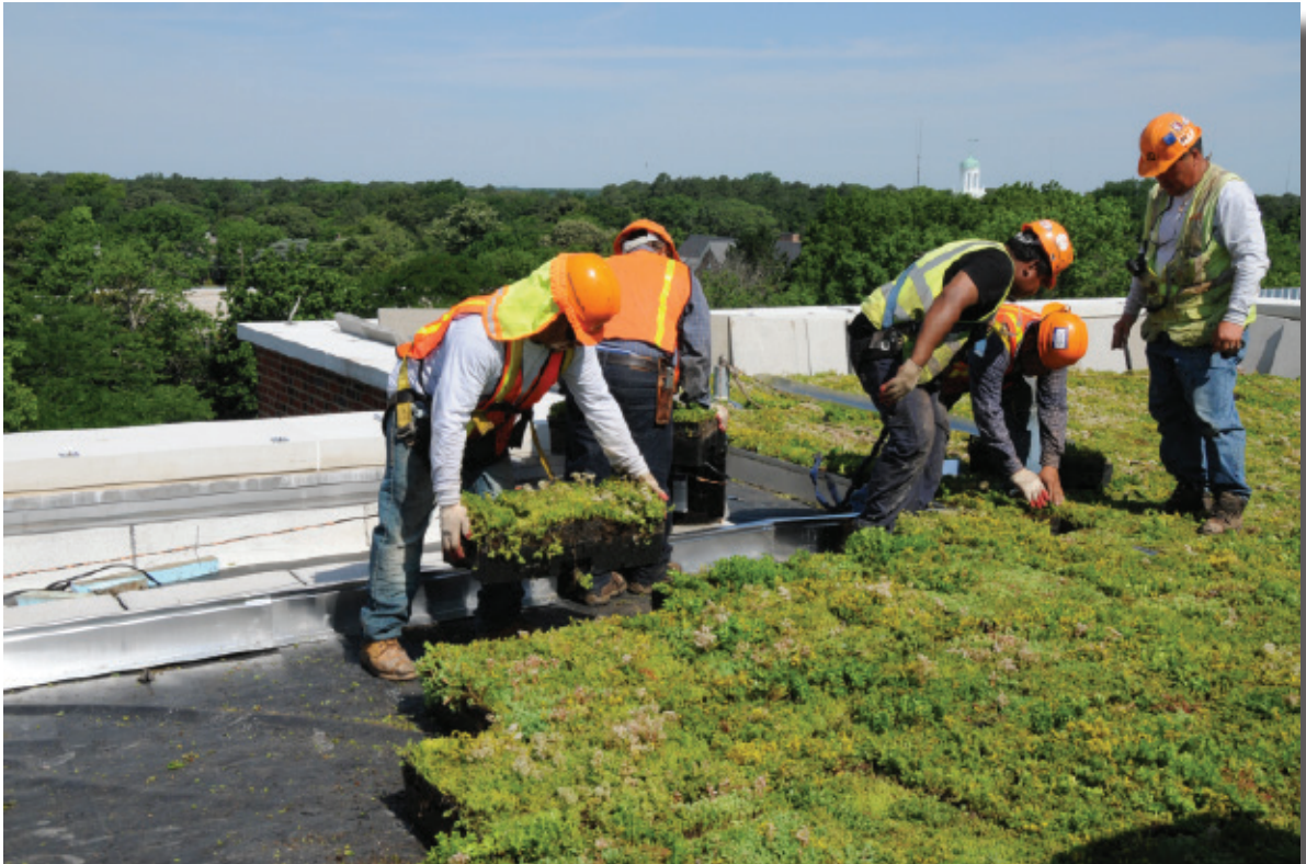
A green roof was installed on top of Salisbury University's Patricia R. Guerrieri Academic Commons, just opened in fall 2016. Comprised of regional plants, it helps with runoff reduction and interior cooling. Image courtesy of Salisbury University.
